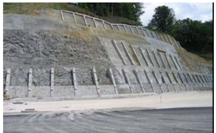
Picture 5: Finale structure and protection of slopes.
